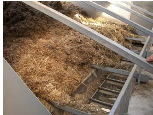
Wood waste is automatically fed to boiler via a 'moving floor'
