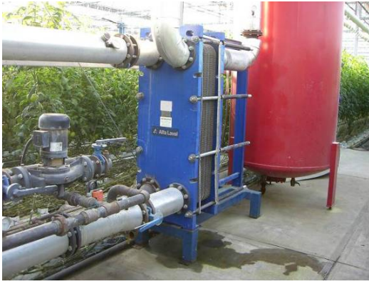
Heat Exchanger to temperate greenhouse irrigation water
